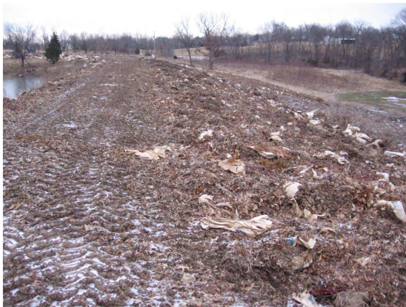
Picture 2. Hillside behind lake dam.
